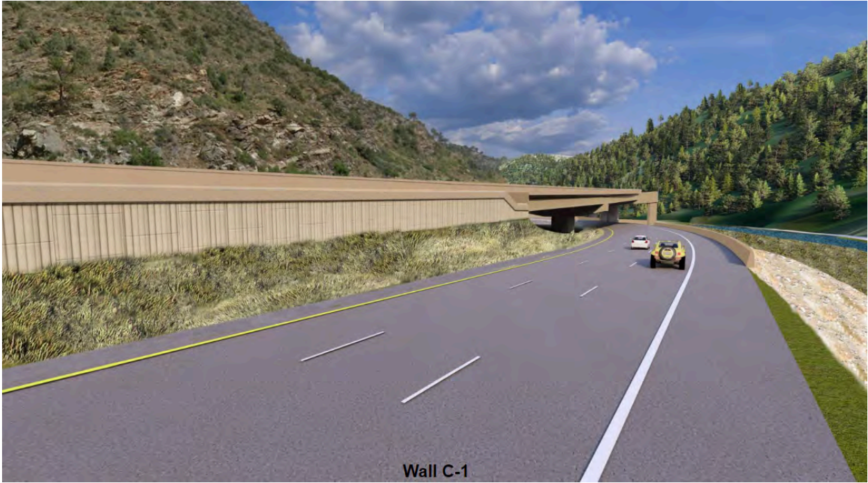
Wall Treatment: 5x5 panels
