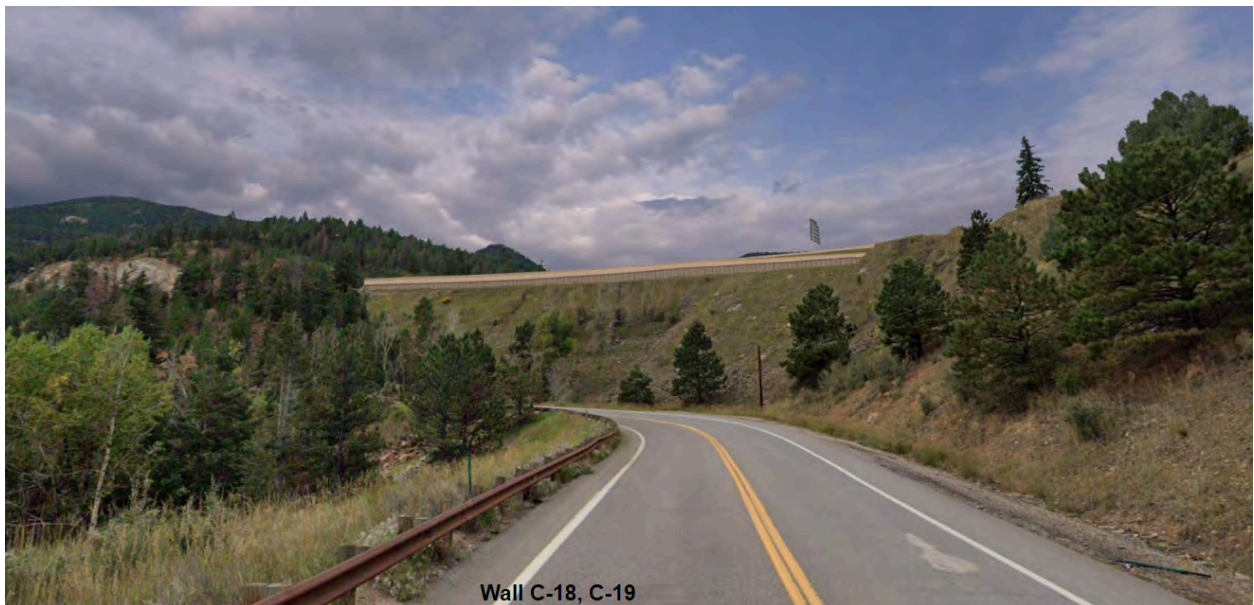
Wall Treatment: 5x5 panels
