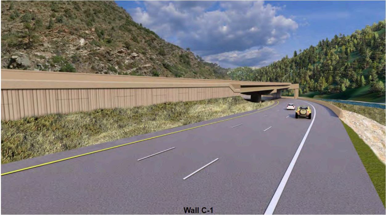
Wall Treatment: 5x10 panels
