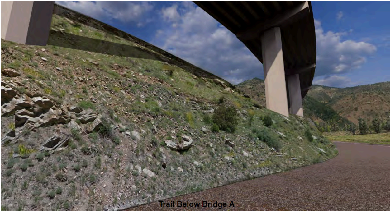
Greenway Trail below Bridge A
