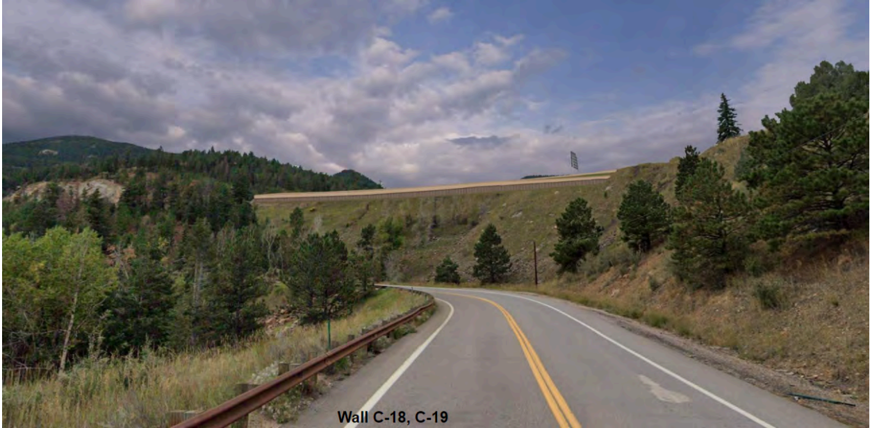
Wall Treatment: 5x10 panels
